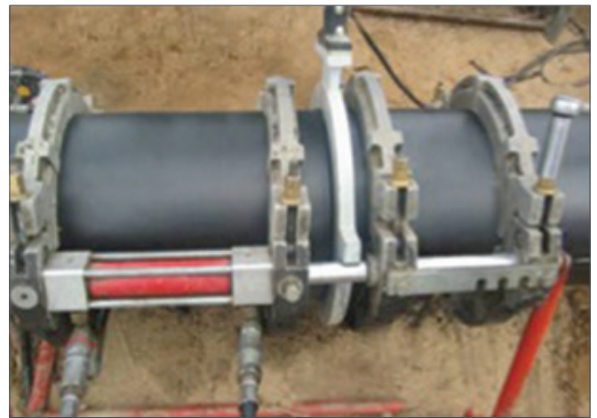
Figure 35a: Re-rounding and Alignment Clamp Assembly used for Wide Bore Pipe
