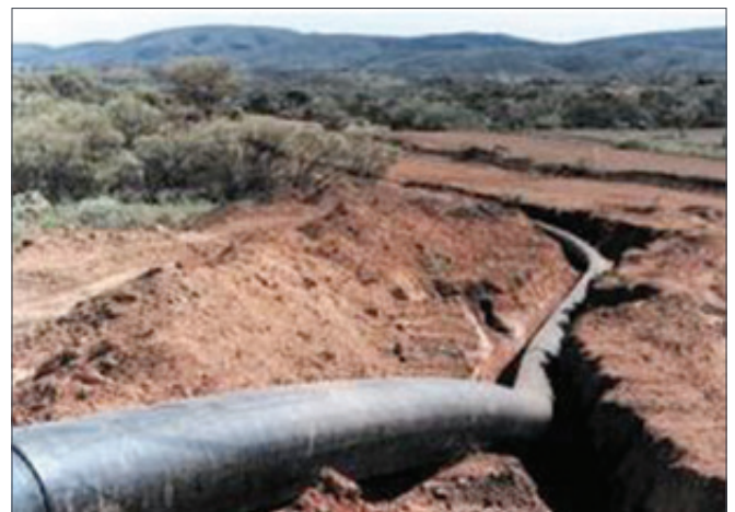
Figure 35b: In-field Laying of Multi-Jointed Pipe
