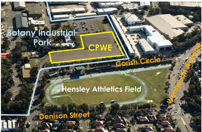
Car Park Waste Encapsulation site to be remediated
